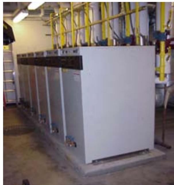
Figure 4. LBNL replaced two boilers with 11 modular boilers to maximize part-load efficiency.
