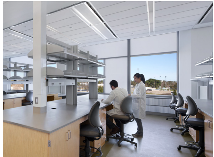
Figure 3. A split window design with distributed internal shading devices, high-reflective interior finishes, and open partitions used at the UC Davis Veterinary Medicine 3B building to enhance access to daylight. Photo: David Wakely Photography.
