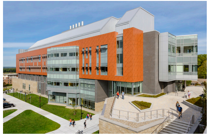
Figure 4. Different sidelighting techniques (curtain wall, punched windows, ribbon windows, exterior shade) in a single façade design by HGA at the University of Rhode Island’s Beupre Center for Chemical and Forensic Sciences. Photo by Anton Grassl; image ©HGA.
