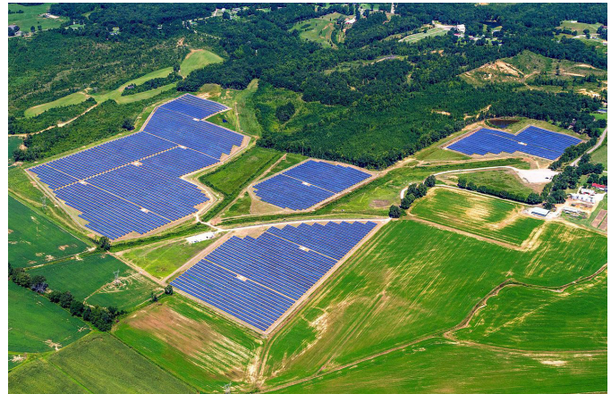
Figure 4. PPAs are often used to fund large renewable energy projects such as this solar farm. Source: Wikimedia Commons.
