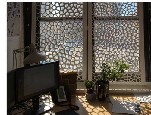
Solar shades mocked up by the architect resemble plant cell structures filter sunlight like the canopy of a forest..
