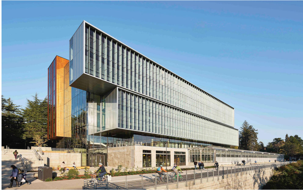
Figure 4. The University of Washington Life Sciences Building (designed by Perkins&Will) used ASHRAE 90.1-2007 as a benchmark during design, showing a 18% reduction in predicted site energy use. The buildings were also benchmarked against the LBT, showing a 59% reduction (153 kBtu/sf/yr vs. a baseline of 370 kBtu/sf/yr). Photo: Kevin Scott
