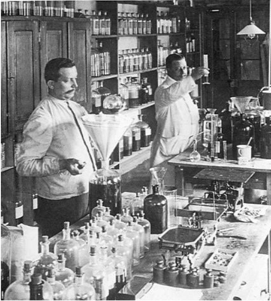
The Kjeldahl process for the determination of nitrogen and protein always was a dirty and very corrosive affair. In this brewery lab from about 1925 the acidic digestion was banned in a wooden fume cupboard located in a side room and separated from the main lab by a glass wall.
