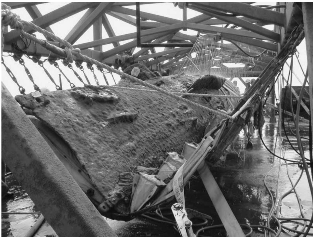
Figure 1. The *H.L. Hunley* on the barge en route to Charleston. Note the 45° angle of the submarine on its starboard side and the spray down system attached to the truss. (Copyright, Friends of the Hunley Inc., 2000)
